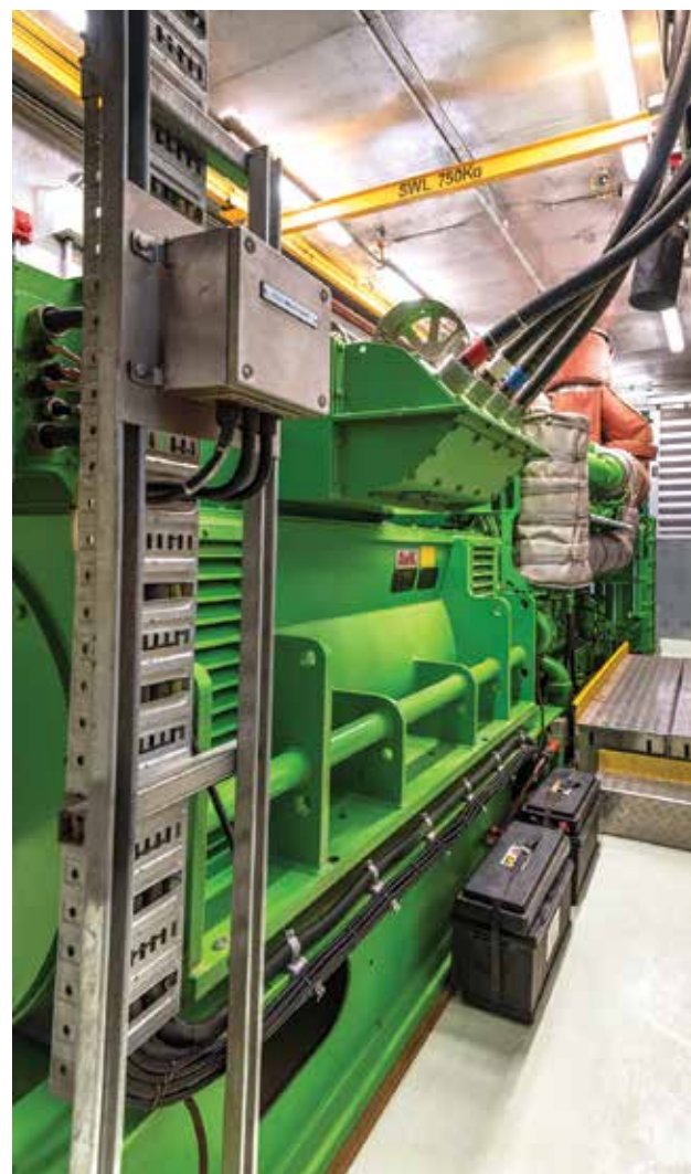
SET 20 JENBACHER (NEW STATION) AT TENNANT CREEK POWER STATION
